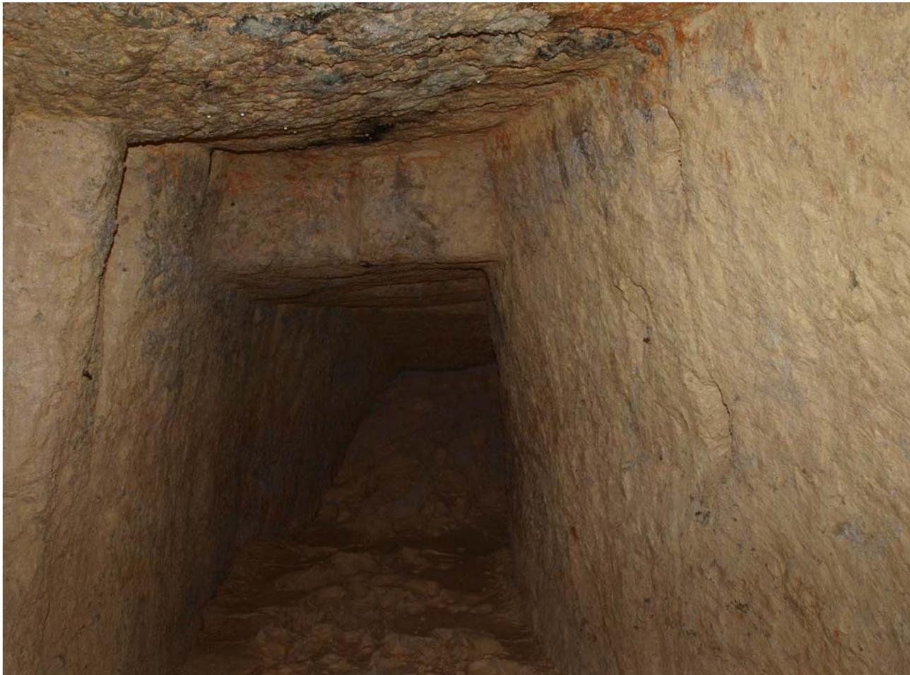
*Fig 11 Roman mine gallery with trapezoidal cross-section in the Cărnic massif.*
