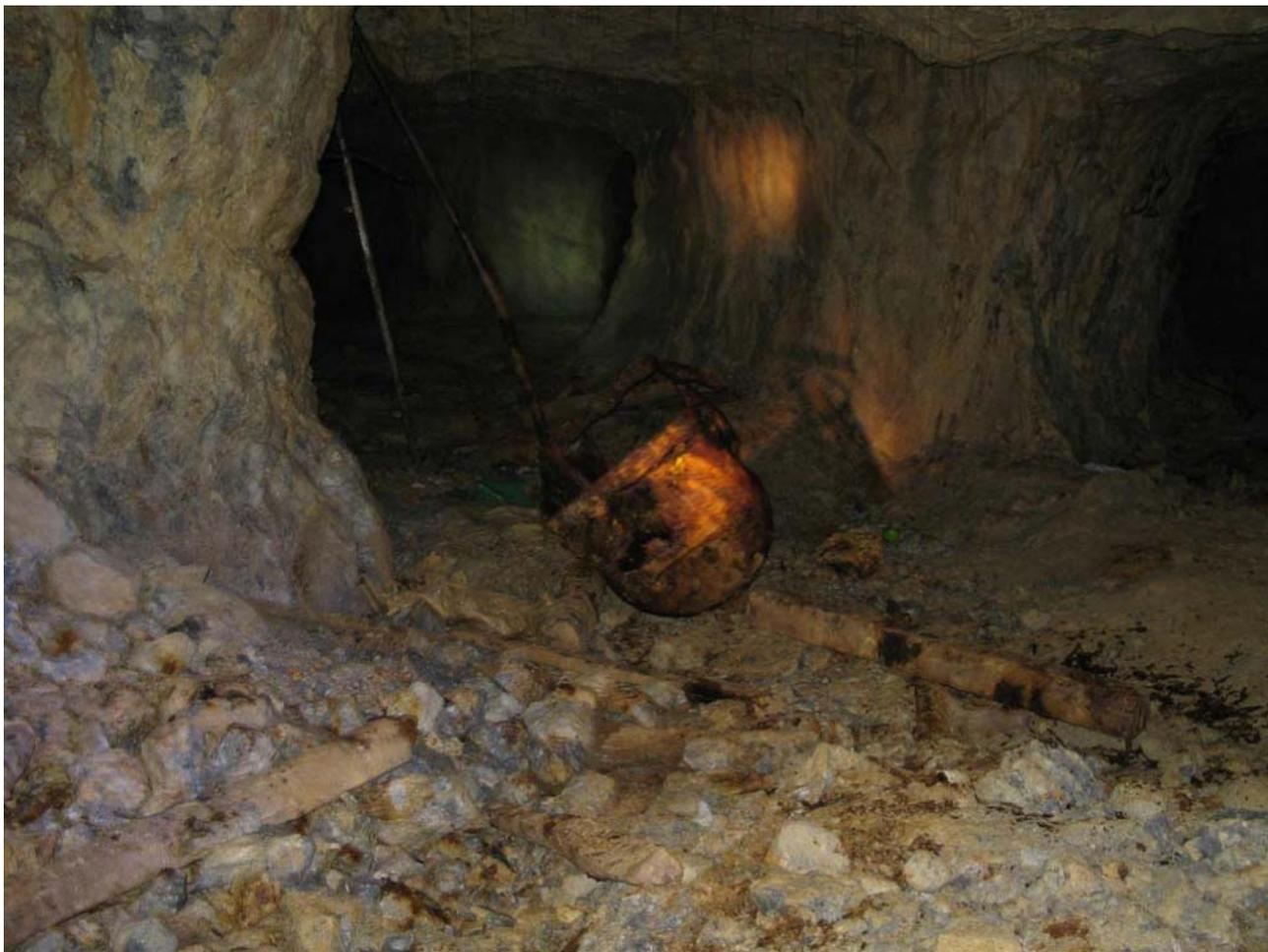
Fig 21 Communist era pillared exploitation chamber in the Cărnic massif.
